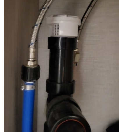
Figure 140. Air admittance valve.
