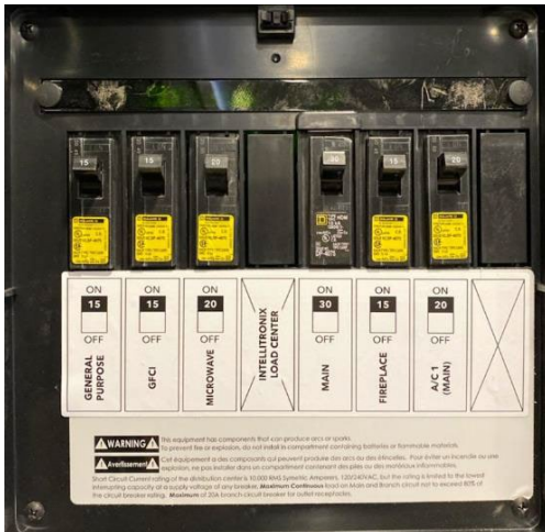
Figure 78. Intellitronix Power Module with 5 circuits installed. The breaker without the yellow label is the input (main) breaker, which would disable all other circuits if turned off.
