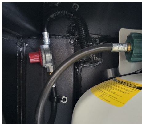
Figure 32. Step down propane regulator for long hose lengths, dropping pressure from tank levels to 30 psi.
