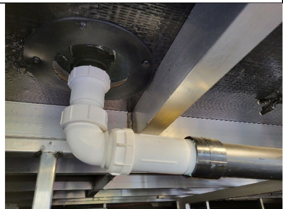
Figure 139. Waterless p-trap under a shower location.
