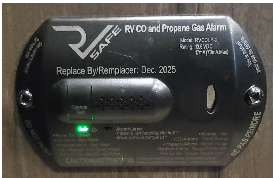
Figure 31. Wall mounted Carbon Monoxide (CO) and Propane alarm. These will be mounted near floor level, usually near stairs.
