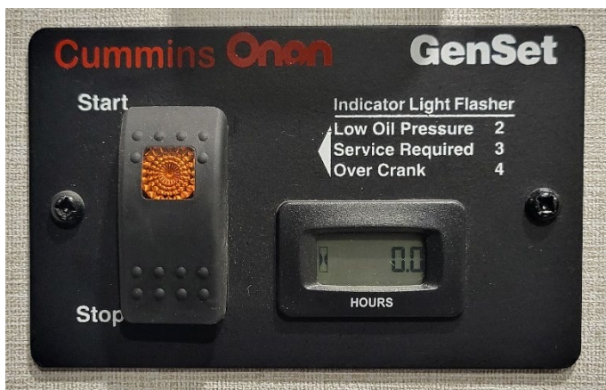
Figure 116. Remote generator start panel. The start/stop button and integrated fault indicator are on the left, and hour meter on the right.
