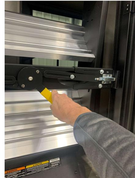
1. Rotate "Latch Handle" to retract the frame latches
